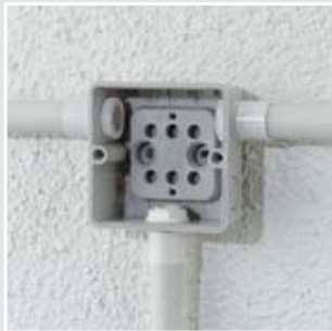
Application: Cable junction box using entries for conduits.
