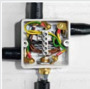
Hensel cable junction boxes with armoured cables according to British Standard.
