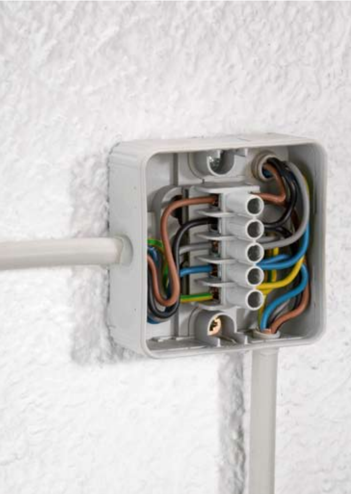
Cable entry from the rear via elastic membranes in the bottom.
