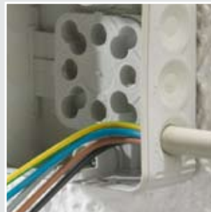
Cable entry via elastic membranes in box walls.
